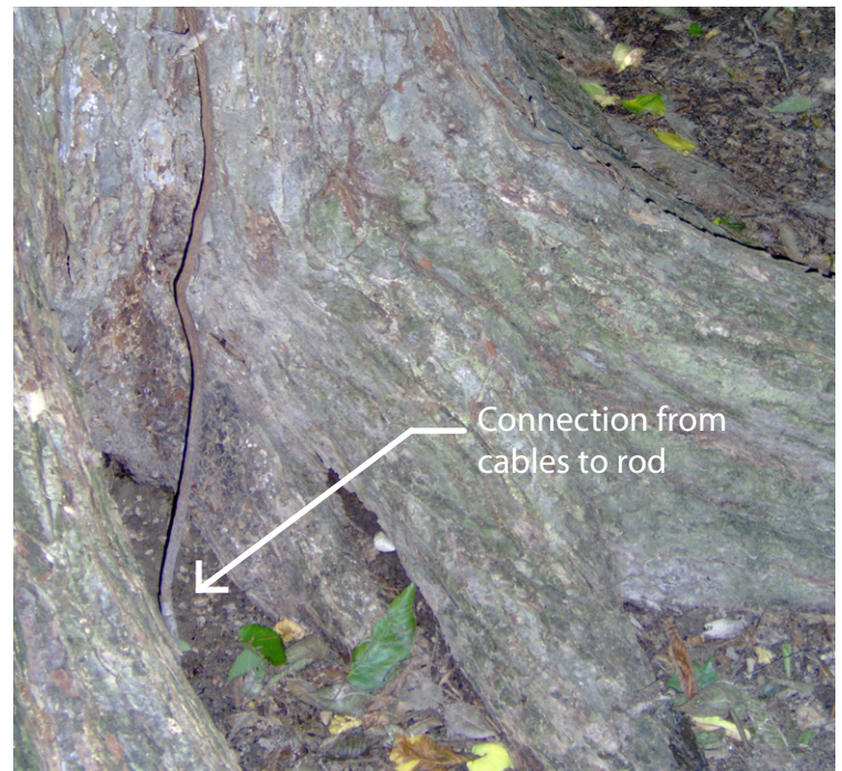
Left: Lightning struck tree. Top: Cable that connects to the underground rod.
